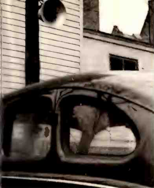
Speaker IIA (see block diagram) operates as "mike" on talk-back from the field to the office.
