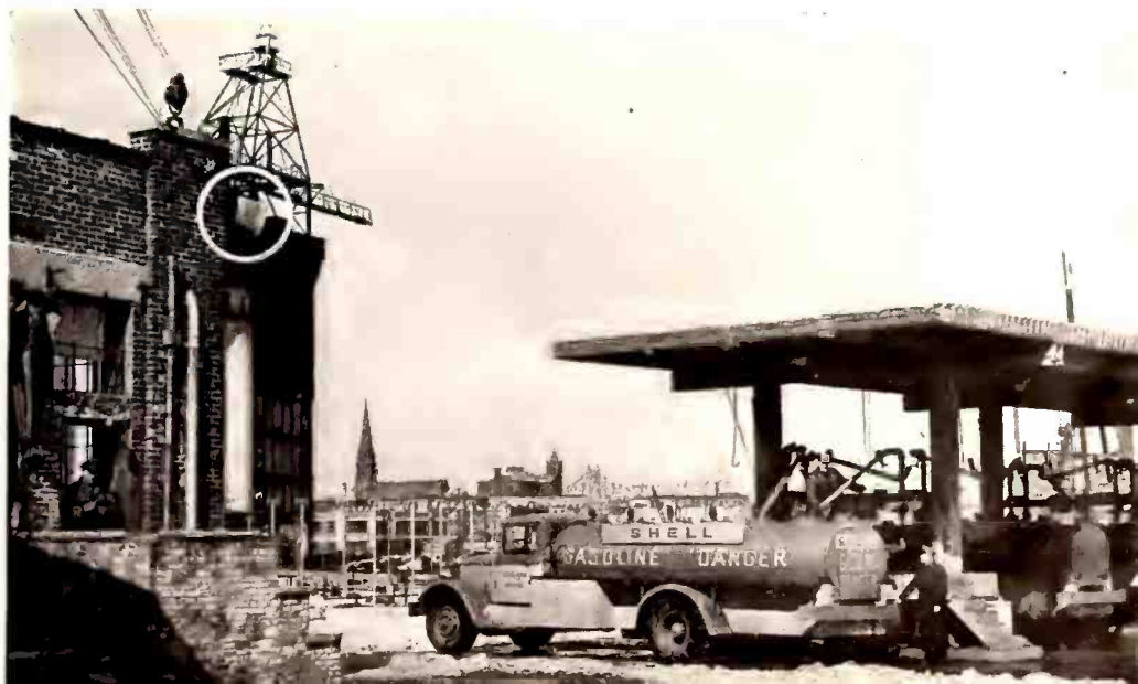
An additional call speaker is mounted over the door to contact office man when he is taking charge of cars in his end of the lot.
