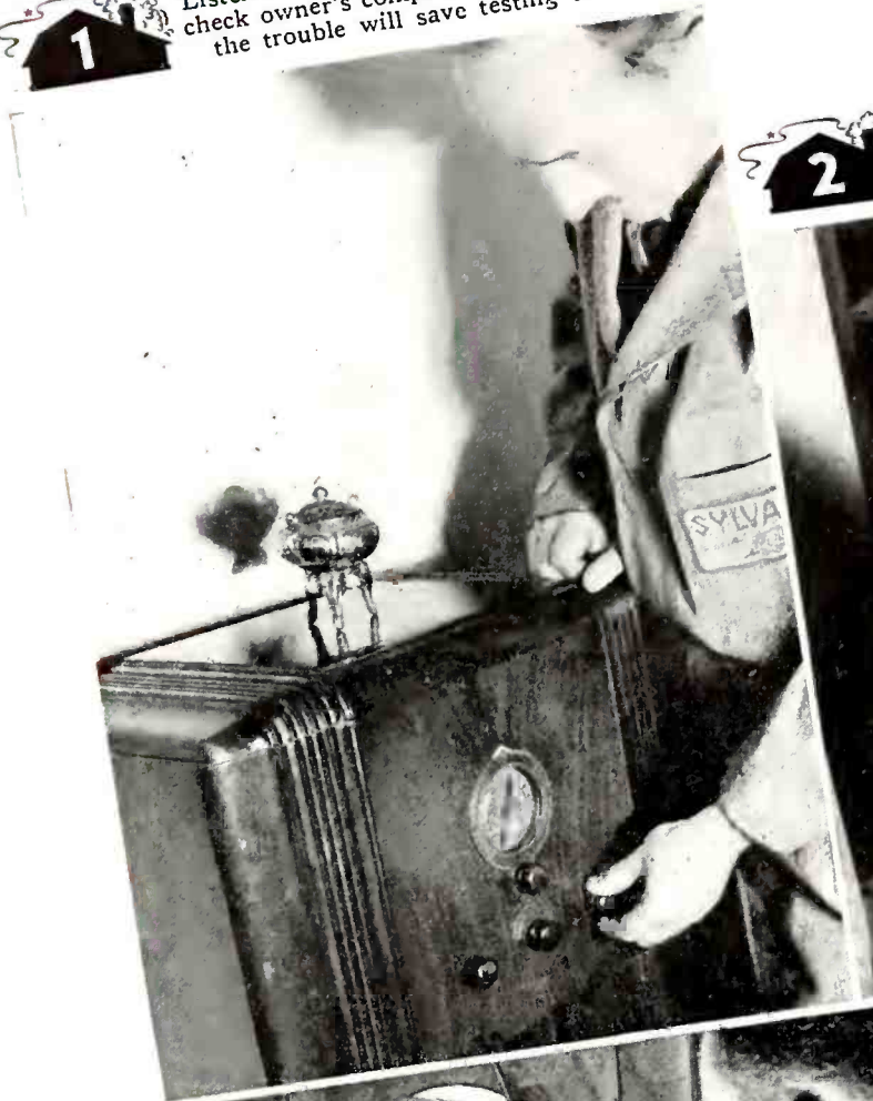
Put down a cover to protect rugs and floor. Test tubes while the owner watches. Weston 778 Serviset used here.
