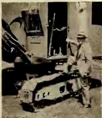
President B. G. Erskine of Hygrade Sylvania, breaking ground for the company's new office building in Emporia, Pa.
