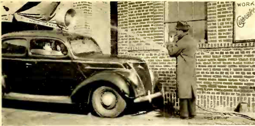
This storm-proof marine type cone speaker made by Atlas Sound is well suited for all outdoor applications. Unit worked okay after rigid test shown above.
