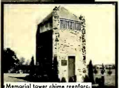
Memorial tower chime reinforcing installation
