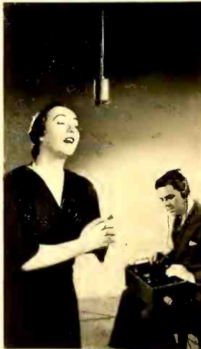
This non-directional Western Electric mike can be made semi-directional by the addition of a small baffle plate.
