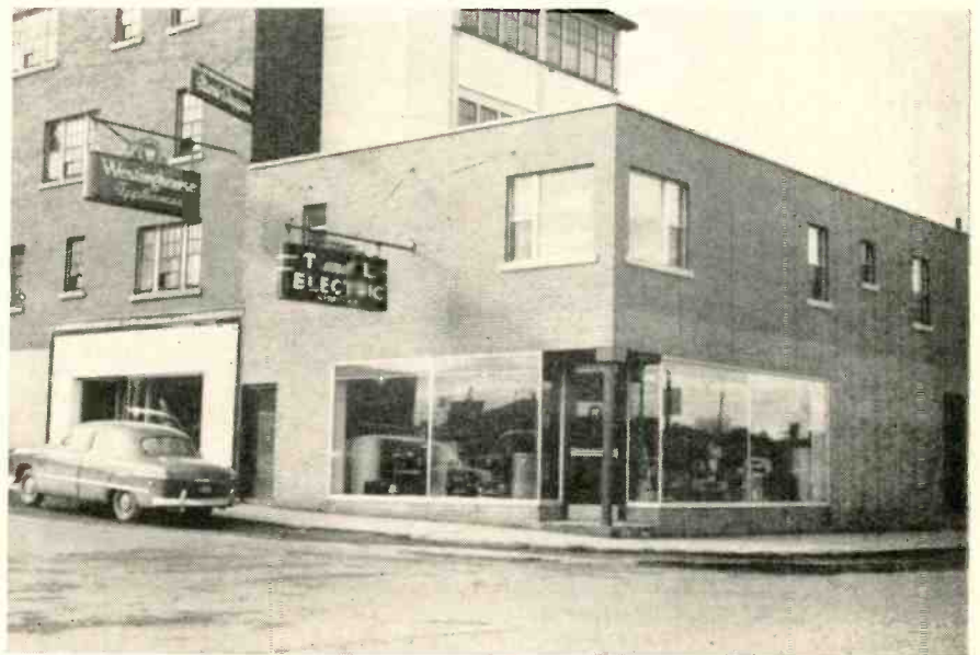
Exterior view of the T and L Electric in Sudbury showing the large area of glass that makes the inside so bright and gives a good view of the merchandise inside. The small store that can be seen immediately behind the car in the left foreground was the location of T and L previous to their present location.
