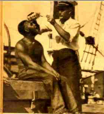
On deck, off Galapagos, the Skipper does some doctoring.
