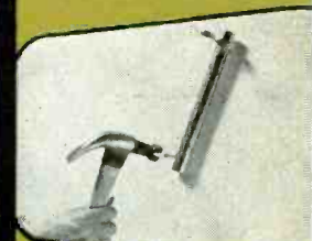
Nail up mounting bracket.
