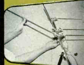
Snap secondary crossarms in place.
