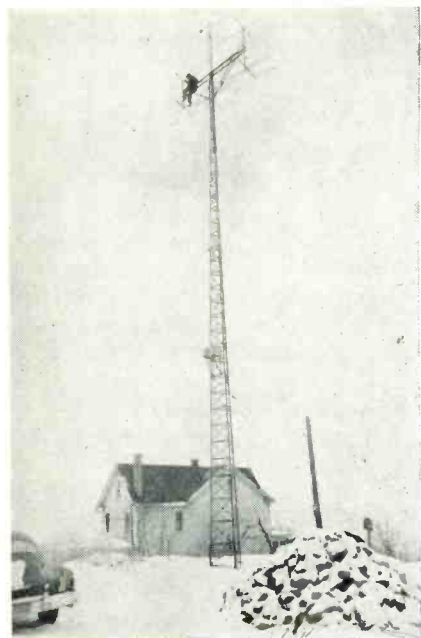
80 ft. tower; antennas mounted on top, and amplifier unit mounted 1/3 the way up the tower.
