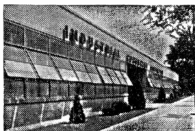
Modern plant built by Industrial Condenser Corp., for manufacturers of Capacitors only.
