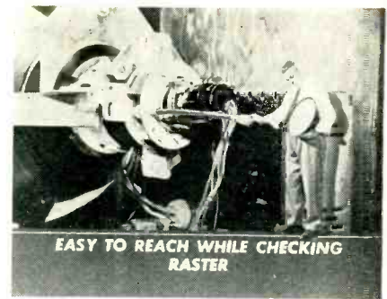
Fig. 6. The provision of an extension on the vernier focus control enables the serviceman to make adjustments while simultaneously checking the raster on the television screen. The vernier control covers a wide range, even under extreme line-voltage variations.
