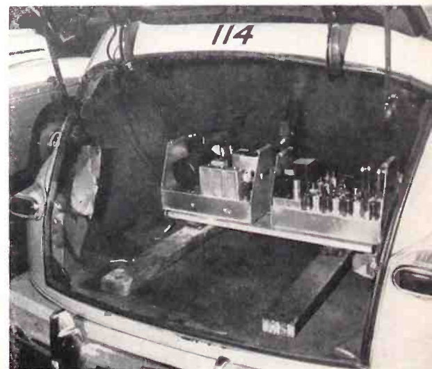
Fig. 2—A typical 25 watt FM mobile transmitter and receiver as installed in a taxi luggage compartment.
