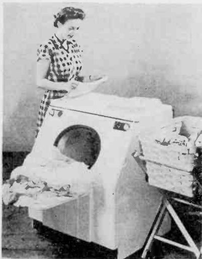
WESTINGHOUSE Automatic clothes dryer. Identical in size and shape to the Laundromat, automatic washing machine, dryer will perform its complete cycle in approximately the same length of time as does the laundromat, thus permitting washing a second load of clothes while the first is being dried. Westinghouse Electric Corp., Electric Appliance Division, Mansfield, O.
