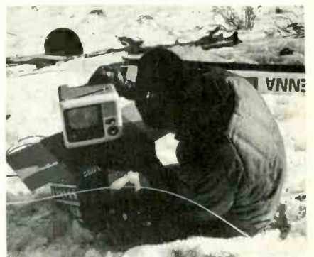
In mountain country, a battery-operated portable TV set should be used to orient the antenna for the best ghost-free pictures.
