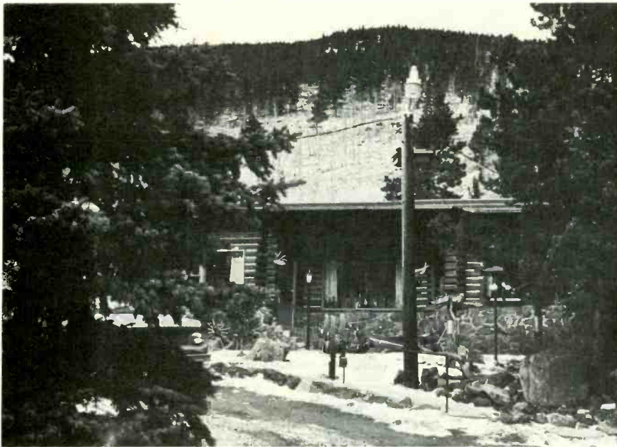
WS-1010 antenna at the top of the hill in the background received all Denver channels, snow-free, from 21 miles away.
