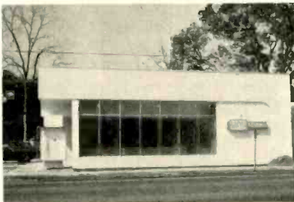
Front view of the nearly completed building shows the minimal window area.
