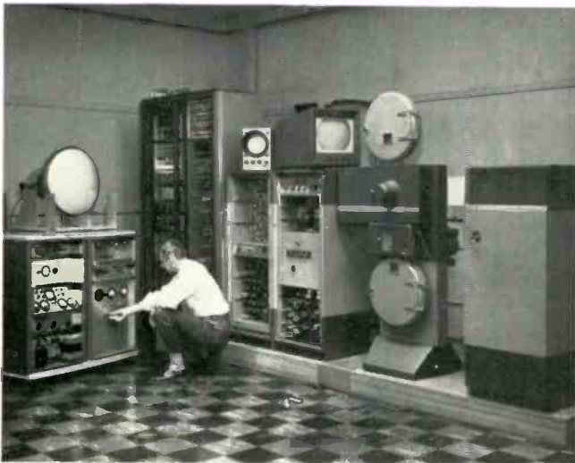
Applications engineer adjusts test equipment to evaluate color CRTs.
