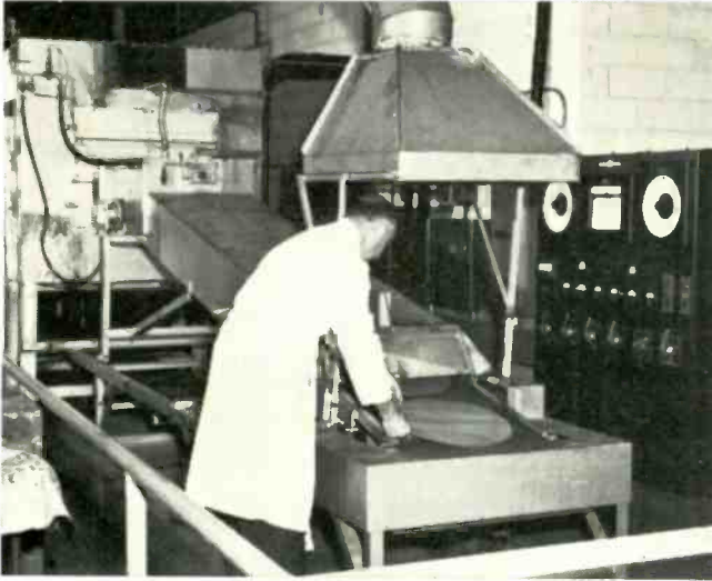
Aperture masks are removed from conveyor after annealing in lehr shown in background....
