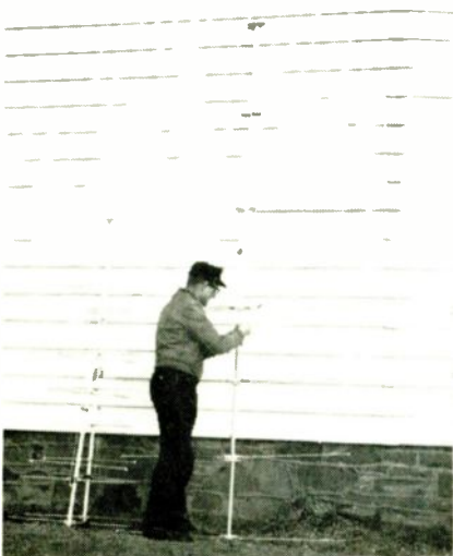
Connecting TACO's low band antenna sections together. Two high band units can be seen to the left. Spring loaded detents on the high band unit allows quick assembly and dis-assembly of the unit.
