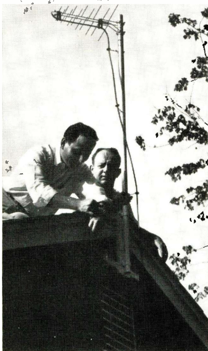
Log periodic type UHF antenna is said to provide uniform gain over entire UHF spectrum.
