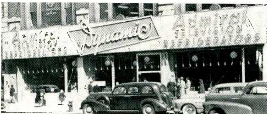
One of the largest and most dramatic neon and incandescent signs ever built tops the new Dynamic Stores' Broadway and 65th Street operation in New York. It has 14 different animations. The interior of the store has been designed to create the effect of three stages, all open and visible from the sidewalk. The front of the store presents an expanse of 75 feet of glass and stainless steel.
