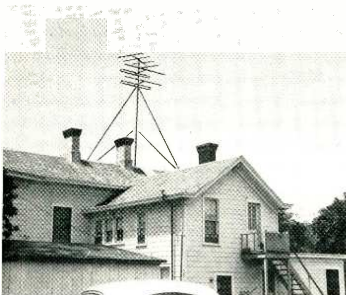
Above and below are typical fringe area antenna installations.
