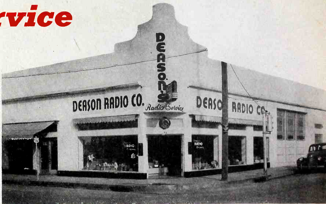
C. G. Deason says that this modern building is practically "the house that service built."
