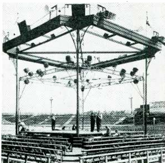
BIG JOB —Here's how the same sound equipment firm handled Madison Square Garden's outdoor bowl for fight fans, placing projectors high up around the lighting support. Lower photo shows control equipment at ringside. Power amplifier was concealed beneath ring
