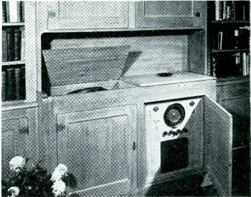
ANOTHER METHOD —It is apparent that careful thought was given this built-in radio installation. It has the air of "belonging" to its surroundings and at the same time the installation provides infinite-baffle
