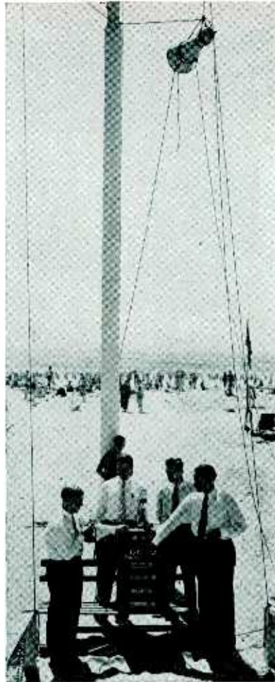
SOUND GOES TO SEA — At Atlantic City, RCA engineers demonstrate a new speaker capable of throwing its voice more than a mile out over the water to bathers, boats. For control of large beach areas sound is a "natural"
