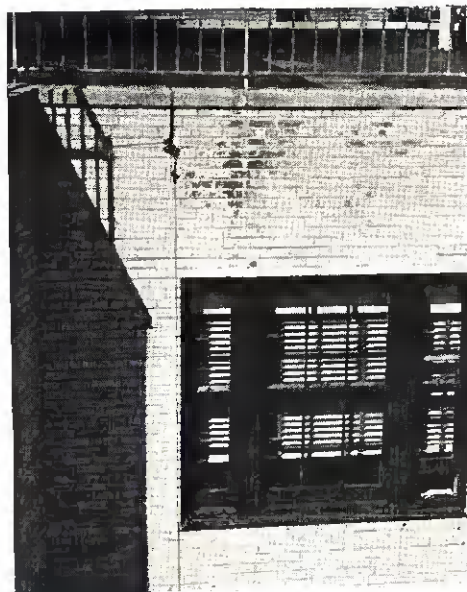
ATTENTION TO DETAIL. — Here's the way a transmission line can be made inconspicuous, running down the side of a large apartment house. Close-up: Note use of flat copper ground-strip to flashing, protected by angle-iron
