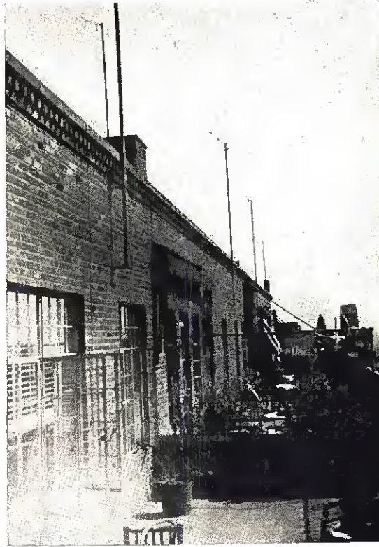
BEFORE AND AFTER —Mystic mazes such as the one shown at the left will one day be banned by law . . . To be superseded by efficient, safe installations such as the one at the right
