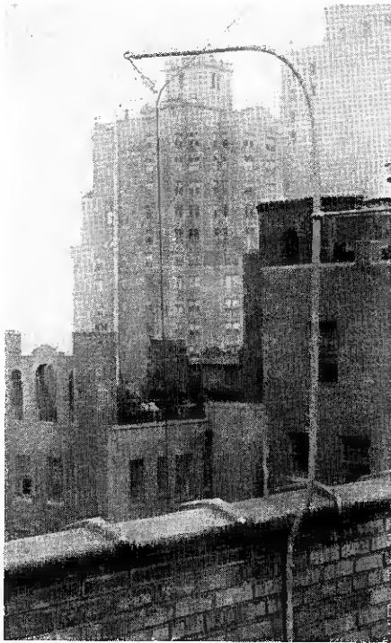
External downleads are usually held away from the coping in this manner
