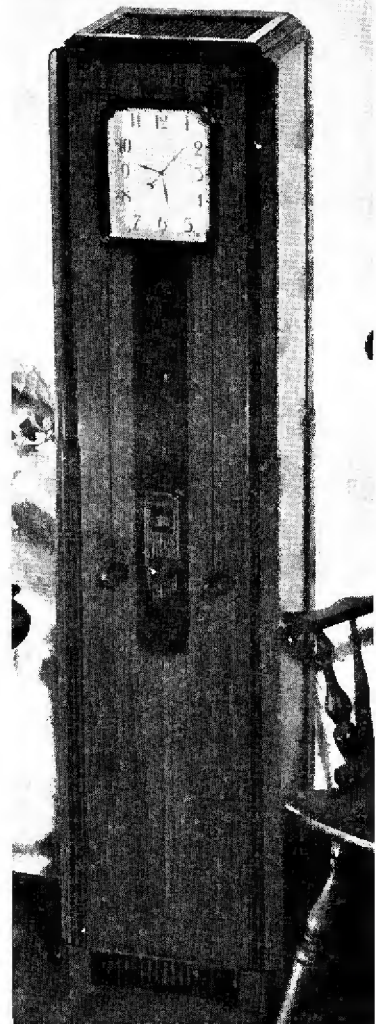
The Columaire Jr. Deluxe—a completely screened 9-tube super-heterodyne set with automatic volume control, fully graduated tone control, Multi-Mu and Push-Pull Power Pentode tubes.
