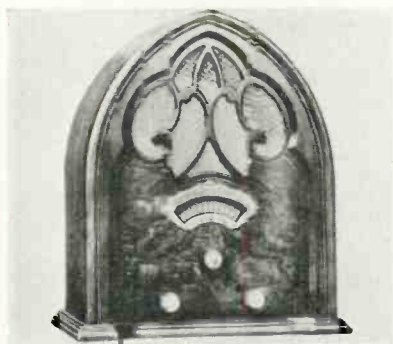
AUDIOLA 610, $48 less tubes T.R.F., with var-mu and pent. tubes
