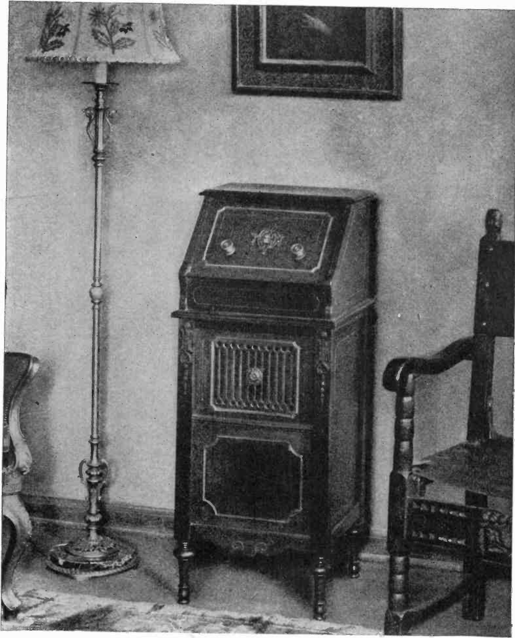
The New Gilfillan Model 20 with Single Dial Control and Shielded Radio Stages.
