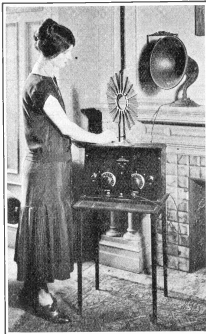
(2) Use a directional loop aerial, adjusting it to the point where the signals are loudest and the static weakest—
