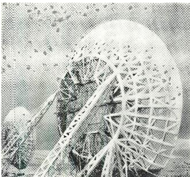
An antenna installation in Arctic Scatter Link. This type of communication is being used extensively during the IGY tests.
