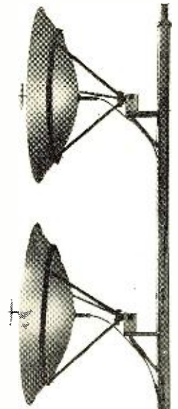
Information relayed by a Mountain Patrolman helps Fire Chiefs plan firefighting strategy and dispatch "cats" and other specialized gear to critical areas. The dish antennas are part of the L.A.F.D. microwave link from Van Nuys base to remote transmitter.
