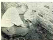
Soldering ground lead
