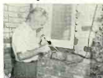
Splicing antenna lead-in
