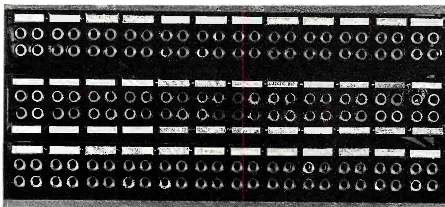
Fig. 6. The three double-jack panels. Jack frames must be grounded to rack.
