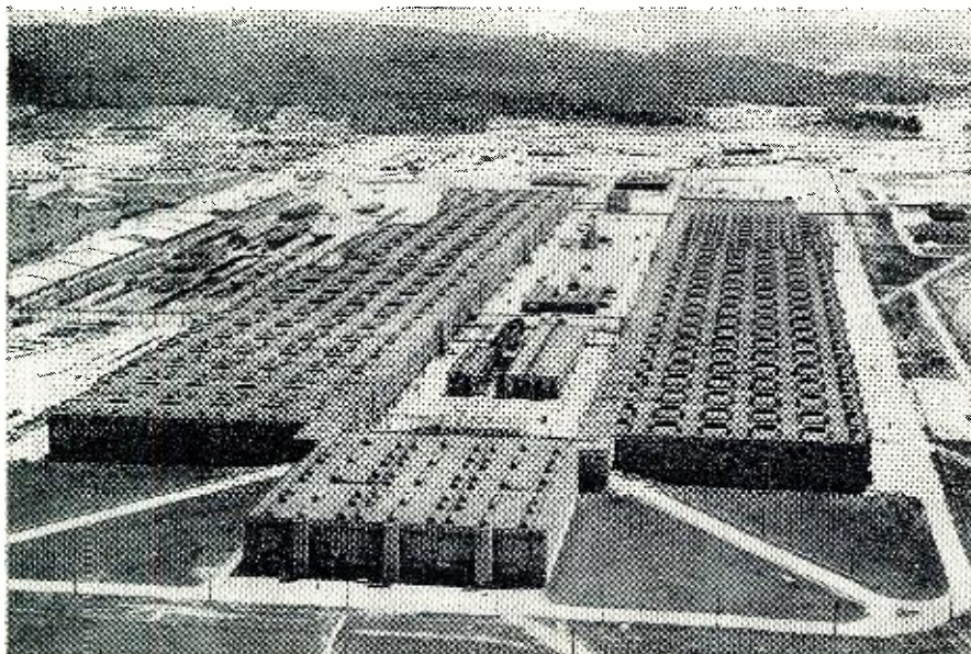
Fig. 7. Gaseous Diffusion Plant at Oak Ridge where ionization gauges play a major role.
