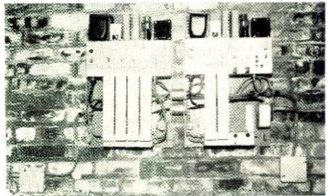
Fig. 9. A typical channel amplifier strip which plugs into the main amplifier unit located near the antenna units.
