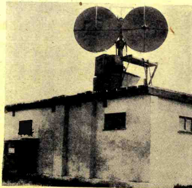
Fig. 3. (Left) One of the seven relay stations in the new microwave system connecting Boston and New York, located atop Jackie Jones Mountain near Haverstraw, N. Y. A pair of shielded lens antennas provides two-way transmission with 1-watt beamed waves at 4000 mc. Developed by Bell Laboratories, the radio relay system provides wide-band communications link for television. Fig. 4. (Right) Parabolic reflector antennas in use with two-way experimental radio relay system for television.
