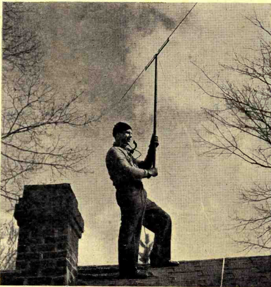
Single dipole used to locate best antenna site. Lead-in connects dipole with receiver where relative signal strength and picture quality is observed for each different roof position of dipole. A portable telephone system provides communication.
