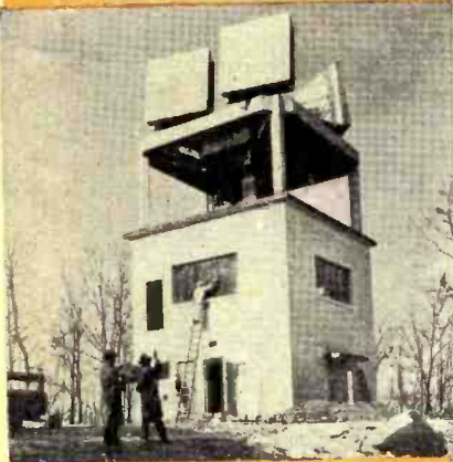
COVER PHOTO: One of A.T.&T.'s experimental radio relay stations linking New York and Boston. Each of these towers will receive television signals and transmit them to next relay—automatically and unattended. Photo by Western Electric
