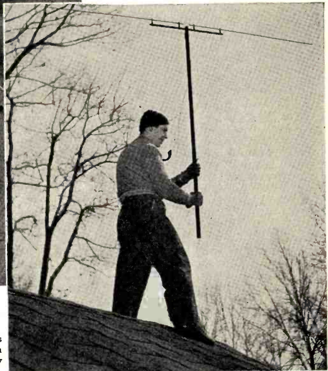
Fig. 2. Portable dipole is used to probe various roof locations for best antenna site. Lead-in connects dipole with television receiver, where relative signal strength and picture quality are observed for each of the various roof positions of dipole.
