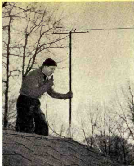
Fig. 6. Before tightening, dipole antenna is oriented for most favorable reception.
