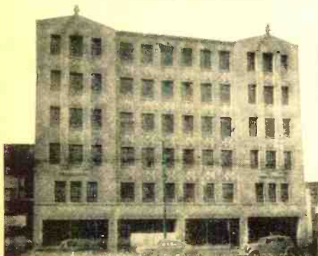
One of Our New Buildings. Air Conditioned the Year Round.
