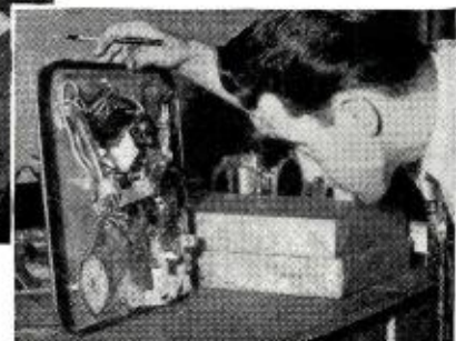
↓ A specialist checks parts functions of a record changer. From the data compiled, "exploded-view" pictorials and repair and adjustment data will be prepared.
