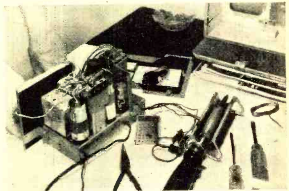
5 Rectifier operation should now be checked by turning the receiver on. The set should operate immediately without the customary warm-up period.
