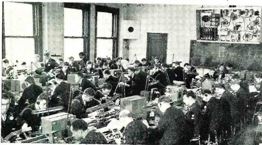
Laboratory where students are building five-tube superheterodynes as one of their projects before graduation. Note the large scale model of the receiver mounted on the wall for the guidance of the students in placing parts.
