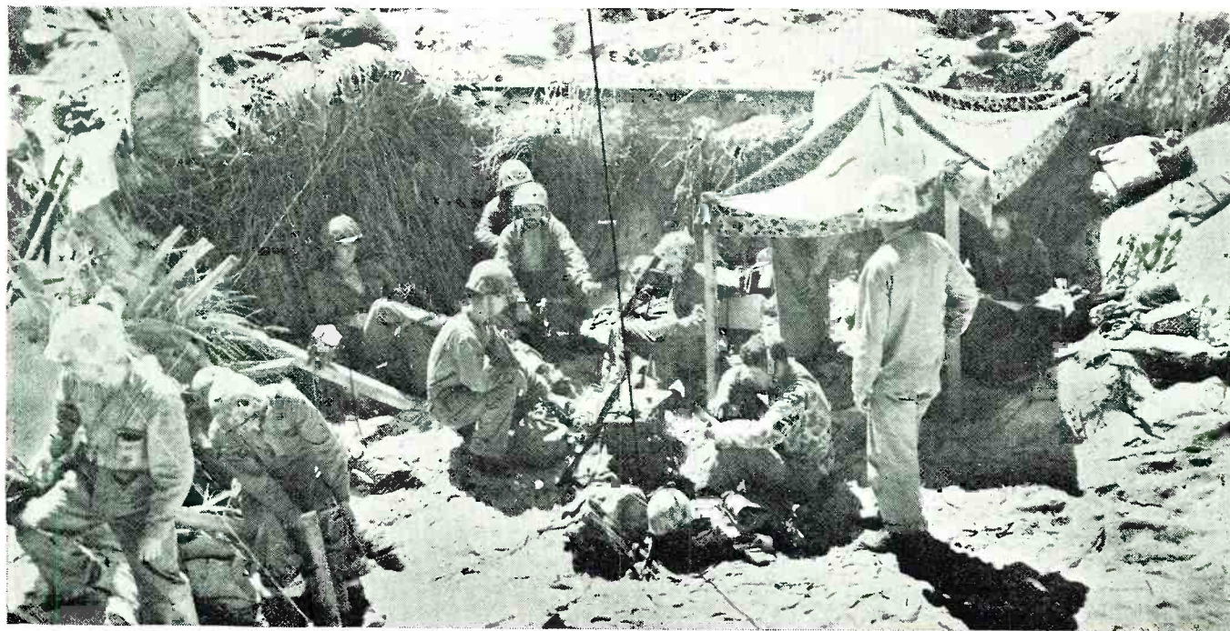
Communications Post of “nerve center” of a Marine Corps regiment on Tarawa. The equipment was set up soon after Yanks landed on the Jap-held island in the face of strong opposition and tough natural barriers.
