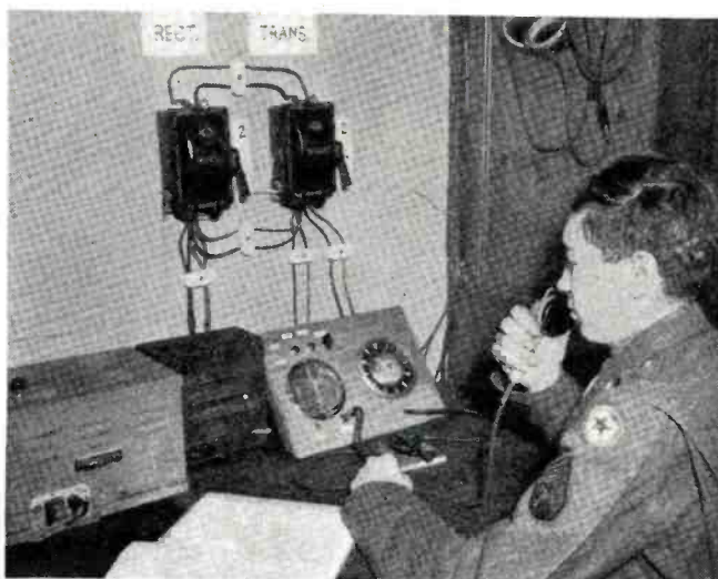
Control station showing receiver and transmitter control panel.
