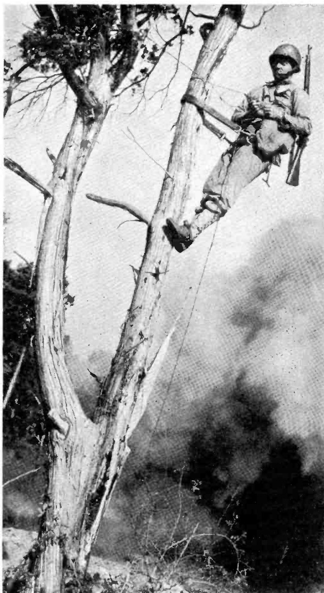
Stringing communication wires during landing operations.
