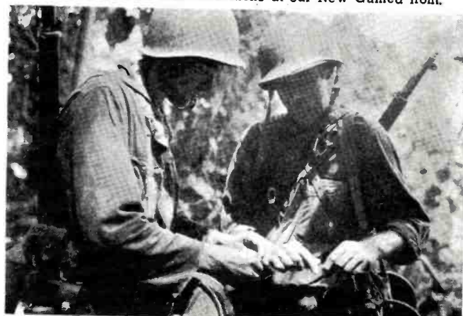
Stringing wire for communications at our New Guinea front.
