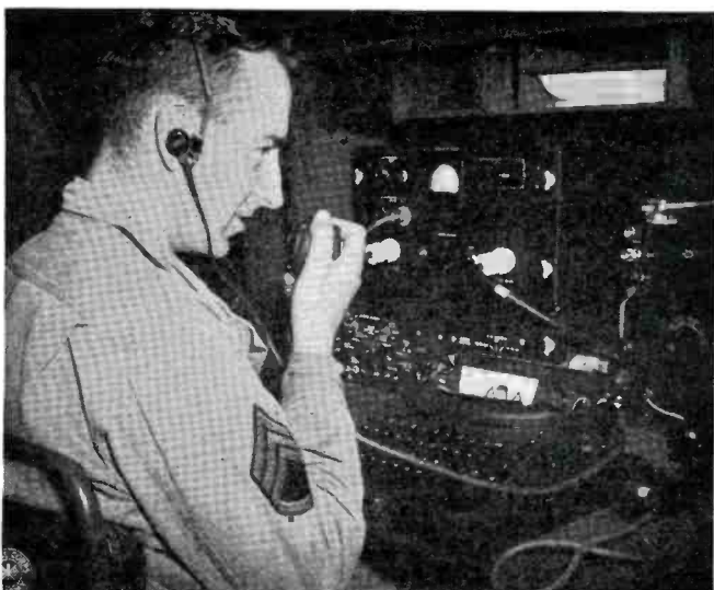
SCR-399 operating position. Operator uses push-to-talk microphone.
