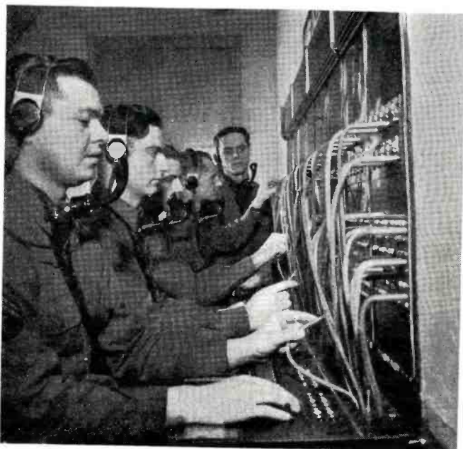
Telephone exchange in Iceland handles 7000 calls a day.
