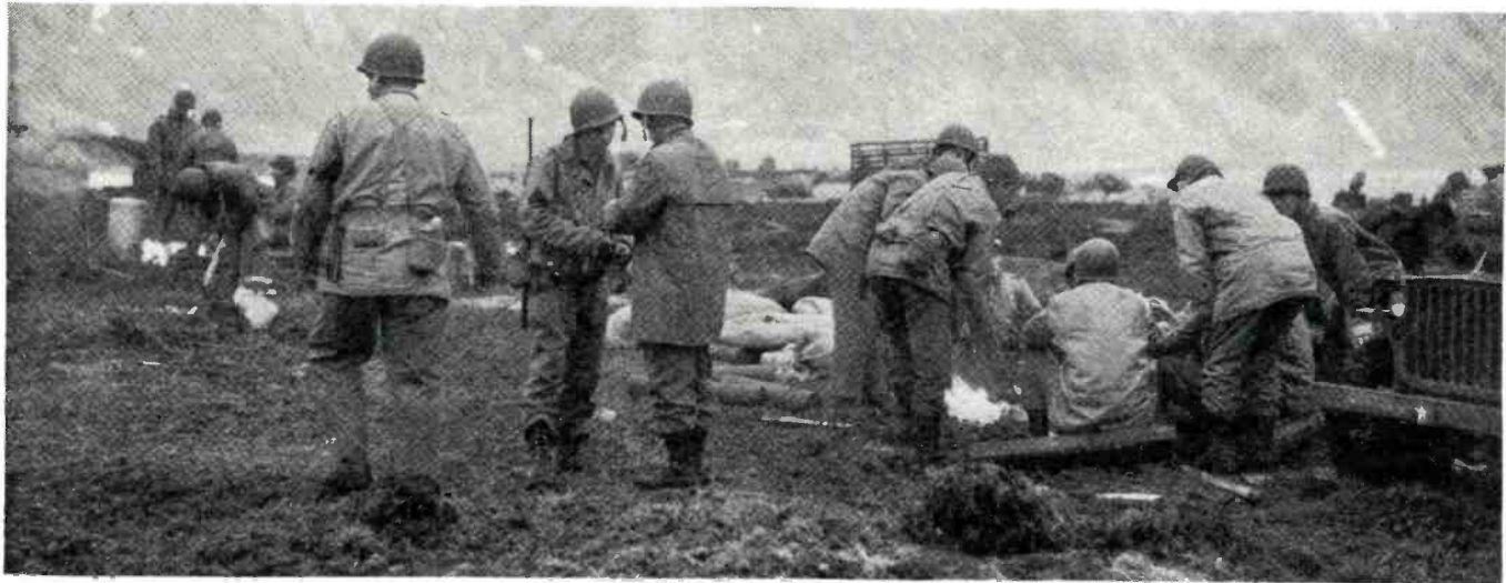
Constructing communication lines—a rather difficult task, considering the rugged Alaskan terrain.
