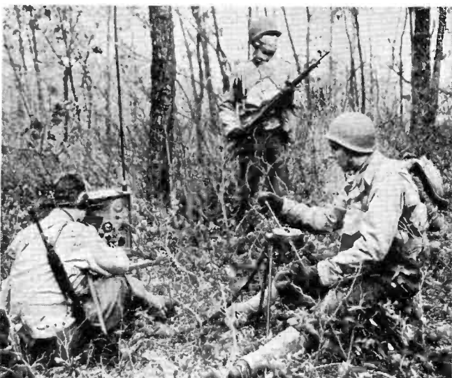
Signal Corps troops with portable hand-generator and receiver.
