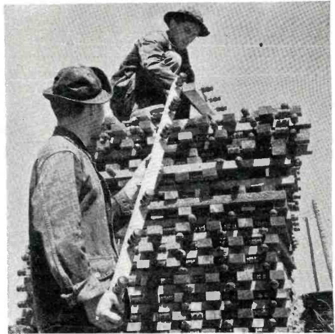
Signal Corps soldiers stacking telephone pole crossarms.
