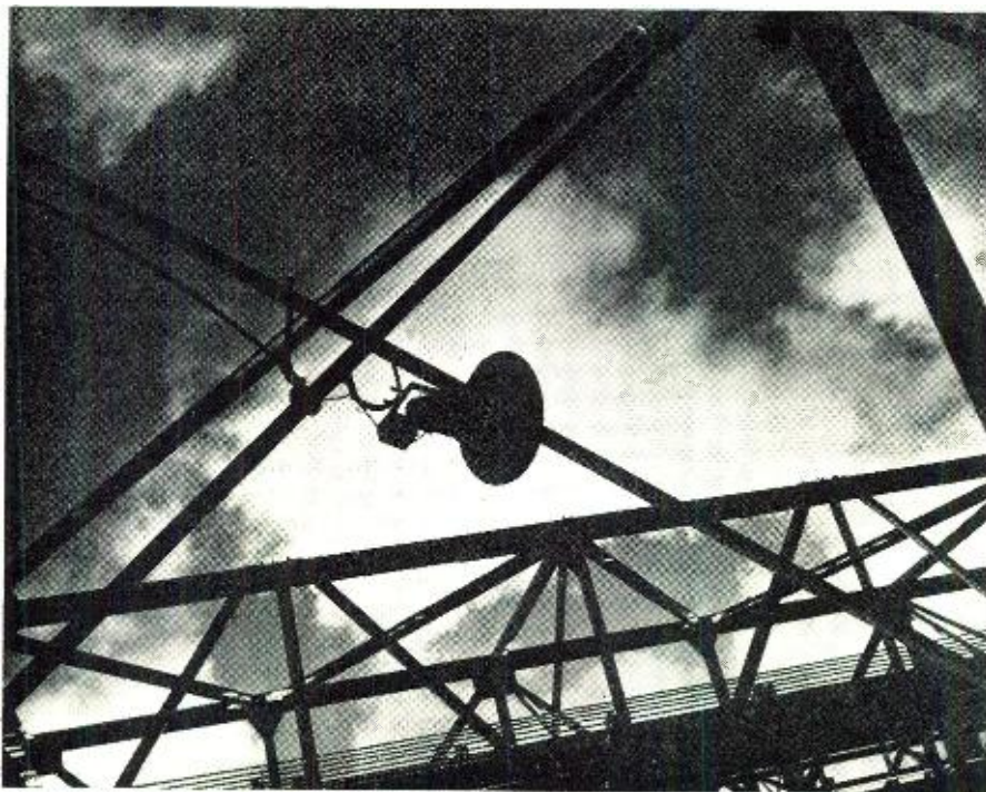
This speaker is installed in the steel framework on ways for new battleship U.S.S. Alabama.
