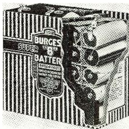
Typical B battery construction.
