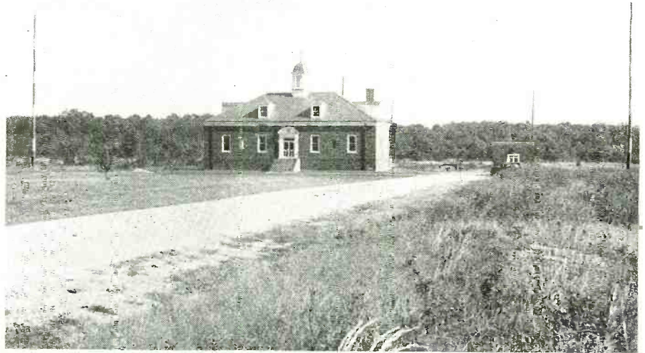
Coast Guard primary radio station. Receiving building and antennae towers.
