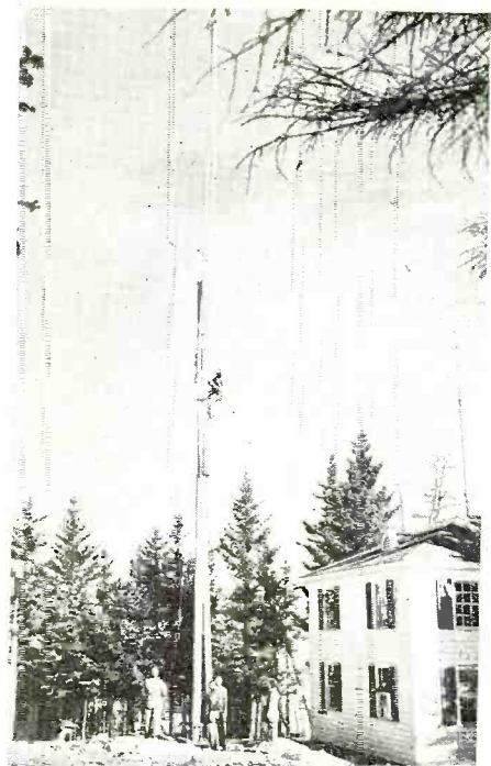
Erecting 75 ft. antenna for NYA station installed at Quoddy Village, Maine site.
