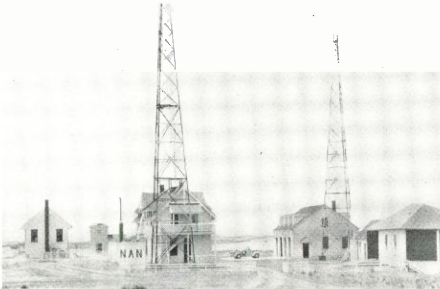
Coast Guard Radio Direction Finder and Lifeboat Station, Cape Lookout, N. C.
