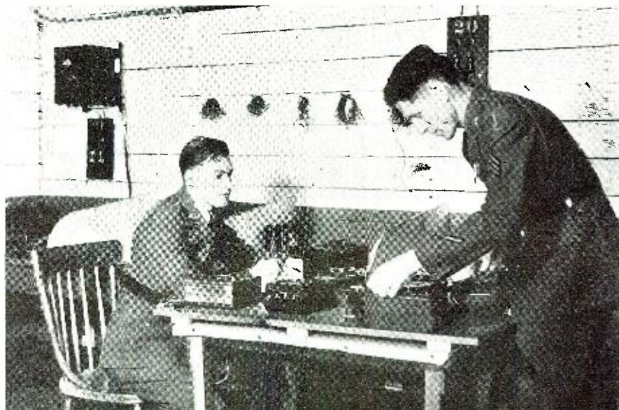
Studying electrical circuits. Note flexible test leads hanging on wall.
