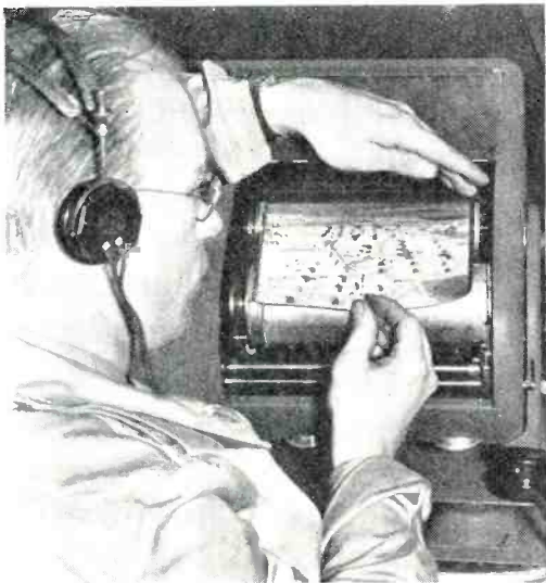
The wet photo of the enemy oil tanks is ready for facsimile transmission as the scout gets okeh signal through his headphones. Photo is clamped onto drum. Scout receives some new instructions while picture is being scanned.
