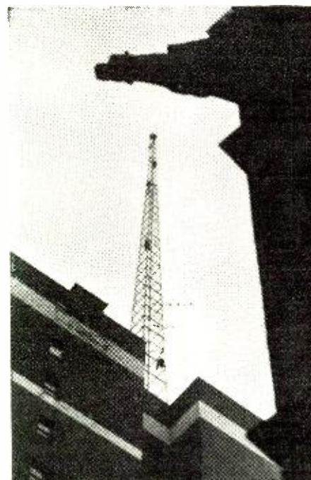
A new tower going up. Notice men working?
