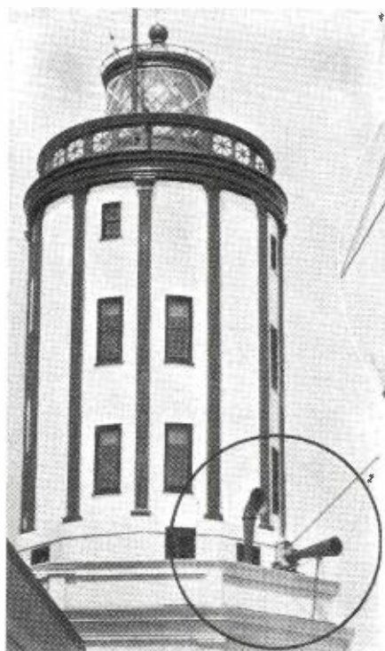
Standing on the bridge, the Captain listens for the fog horns (inset). Noting the time difference between them and the simultaneously sent radio signal, he computes position.
