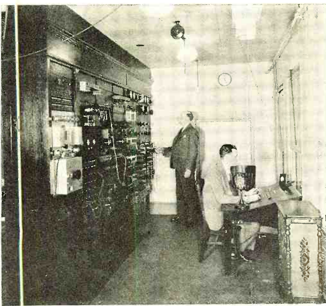
CONTROL ROOM OF TIMES SQUARE STUDIO
